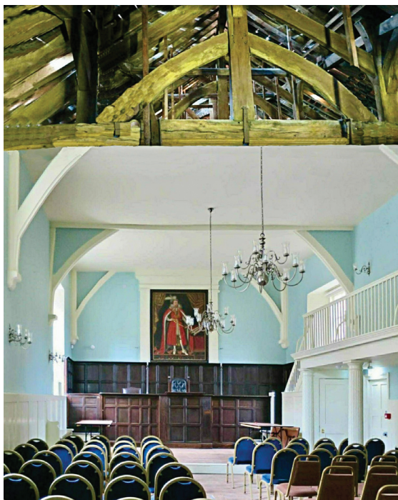
FIG. 244 – Bury St Edmunds Guildhall: Composite view with roof of AD 1376–7 superimposed above ceiling of the Court Room ( photo: Bob Carr ).
